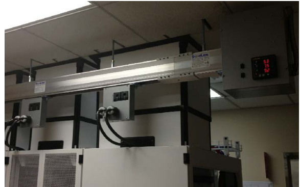
Starline IDF installation example
